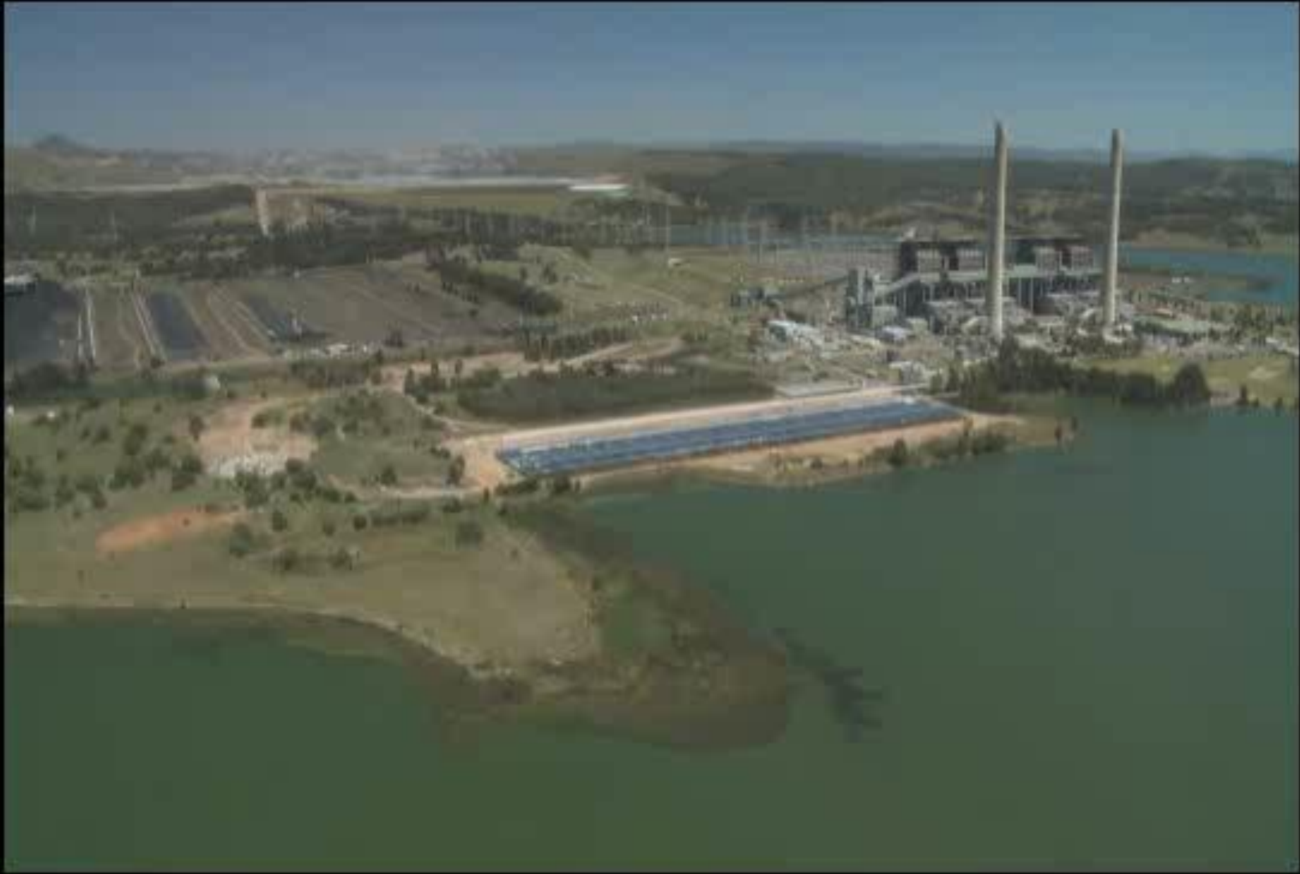
Source: Macquarie Generation http://www.ausramediroom.com/download/LiddelSolarThermal_17Nov09_MPEG-4-1280x720.mp4.zip
